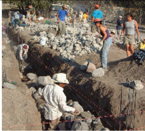
Figure 21: Building zapatas
