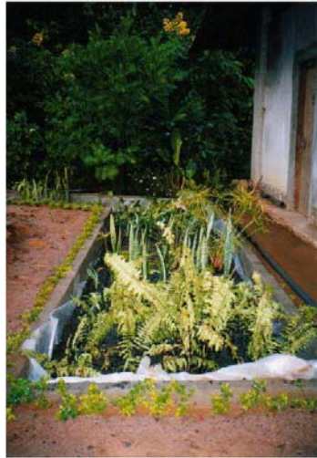
Figure 26: The vertical flow planted gravel filter unit of the Swiss Residence Hotel after commissioning
