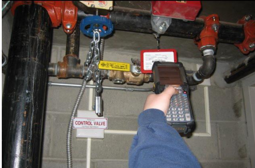
Inspection of Sprinkler System
