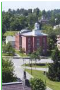
View of Pomeroy Hall from the Old Mill Tower
