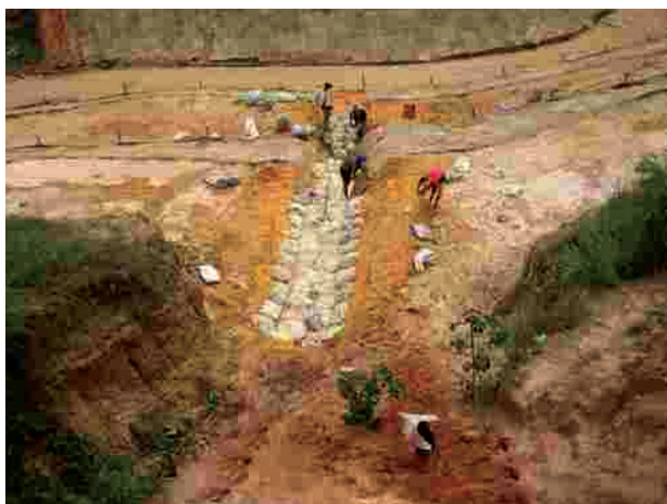
Figure 6 Gullied area in São Luis Municipality, Maranhão State, during rehabilitation work .Photo by Jose Fernando Rodrigues Bezerra.
