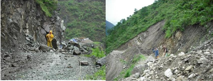
**Figure 2.** The highest landslide erosion occurred along a 1 yr old road (DXD) leading to a remote village and a future hydropower plant just south of Daxingdi, Yunnan, China.
