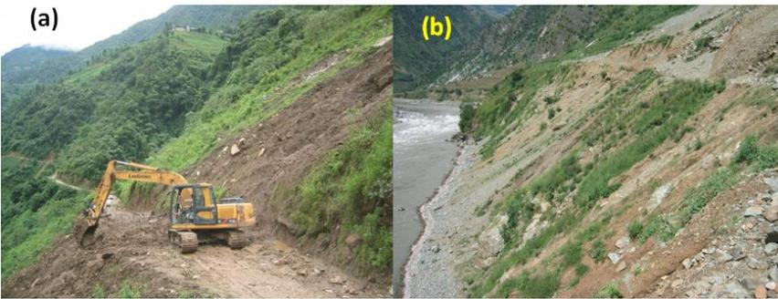
**Figure 7.** (a) A section of the FG2 road several kilometers north of Fugong that was temporarily closed by a landslide; and (b) secondary road to a small mountain village near Daxingdi (not included in our landslide survey) that was abandoned during construction because of excessive landslides.
