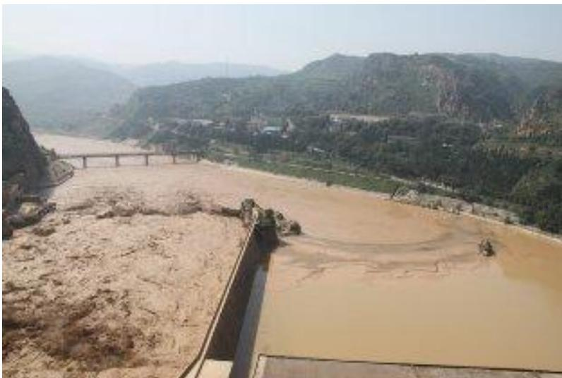
In this photo, the Sanmenxia Power Plant is not generating electricity, but discharging sediment.
