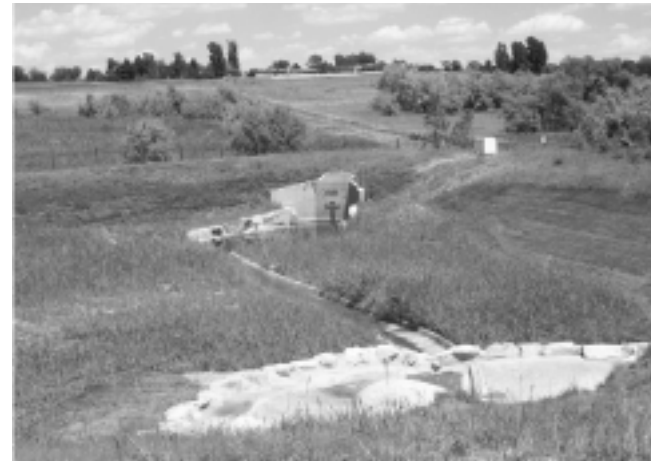
Figure 4. After Modifications Healthy Grass Provides a More Attractive and Maintainable Bottom. Note sedimentation forebay and inlet in the foreground. [Photograph used with permission of Wright Water Engineers, Inc. (WWE).]
