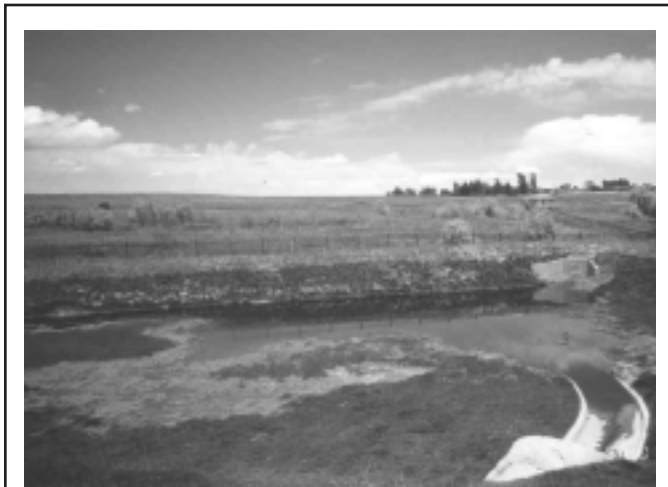
Figure 1. Before Modification Long-Term Inundation Killed the Sod Planted in the Bottom of the EDB and Created Boggy Conditions. [Photograph used with permission of Wright Water Engineers, Inc. (WWE).]
