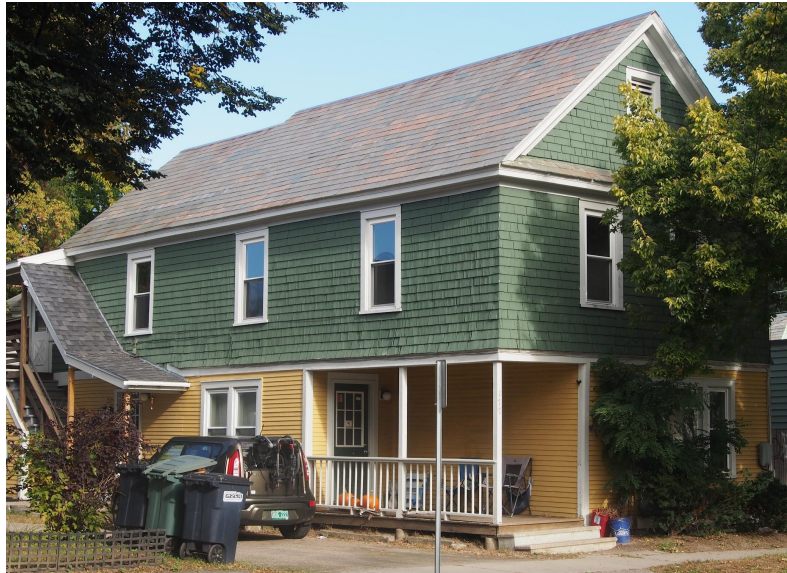
Fig. 10. View of the Mintzer House as it stands today.
