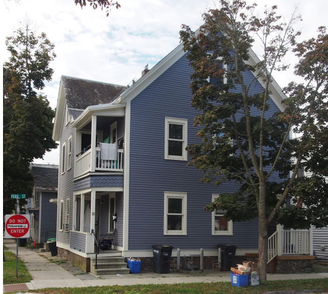
Fig. 6.View of the Apartment Building at 27 & 31 Peru Street as it stands today.
