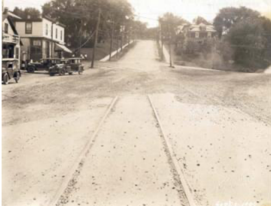
Figure 3. Colchester Avenue at Mill Street, showing the 485 Colchester Ave grocery store and entrance to Barrett Street in the top left, September 1929, facing south. Photograph by L.L. McAllister, courtesy of UVM Special Collections.
