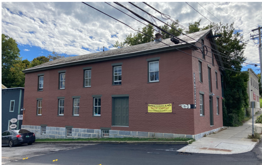
Figure 4. North elevation of the Duncan Blacksmith Shop building, October 2022, facing south. Photograph by Lucas Newton.
