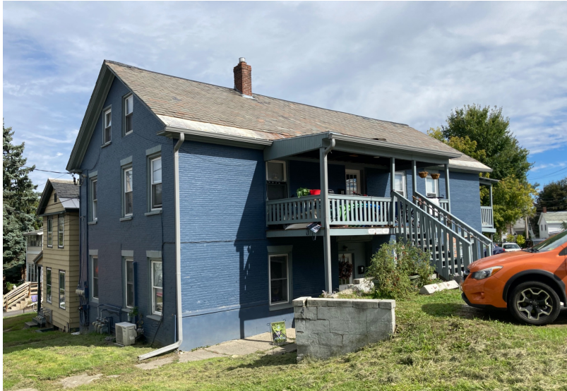
Figure 9. South elevation (right) of 6 Chase Street, October 2022, facing northeast. Photograph by Lucas Newton.
