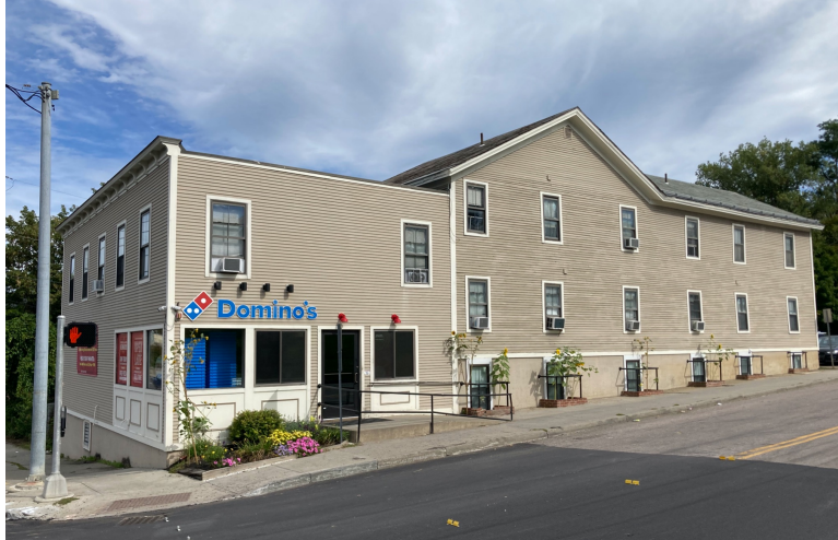
Figure 2. South elevation of the Hickock-Burlington Cotton Company Tenement building, October 2022, facing northeast. Photograph by Lucas Newton.
