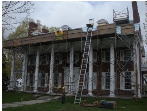
Renovations to the building in 2011.
