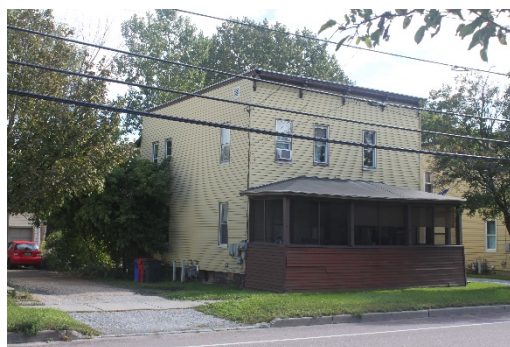
Figure 15 – 112 North Avenue, ¾ record shot. View facing southeast, photo taken by author, 9/26/2022.
