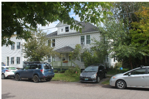
Figure 29 – 22-24 Drew Street, primary façade. View facing northeast, photo taken by author, 9/26/2022.
