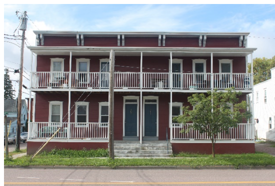
Figure 8 – 103-105 North Avenue, primary façade, view facing west. Photo by author, 9/26/2022
