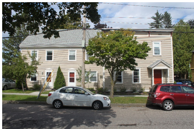
Figure 25 – Façade of 8 Strong Street. View facing north, photo taken by author, 9/26/2022.
