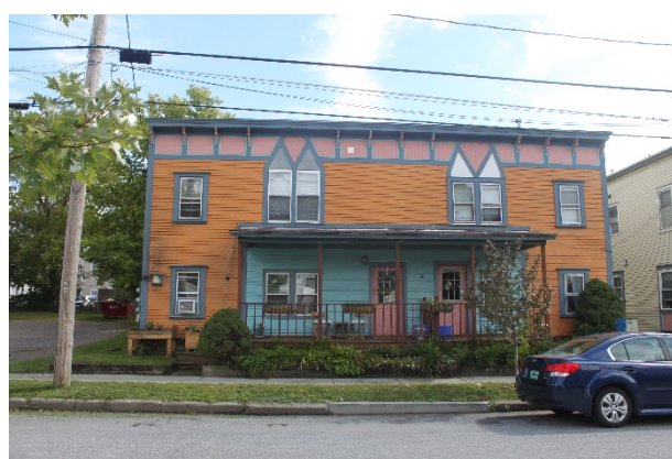
Figure 22 – Primary façade of 88 Pitkin Street. View facing east, photo taken by author, 9/26/2022.
