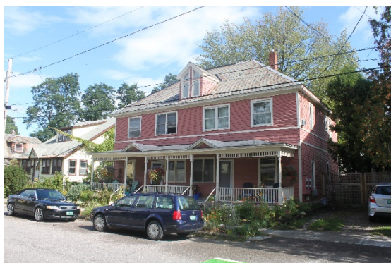
Figure 19 – 72 Lakeview Terrace, view facing northeast. Photo taken by author, 9/26/2022
