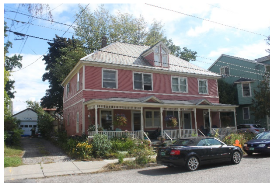
Figure 20 – 72 Lakeview Terrace, view facing southeast. Photo taken by author, 9/26/2022.
