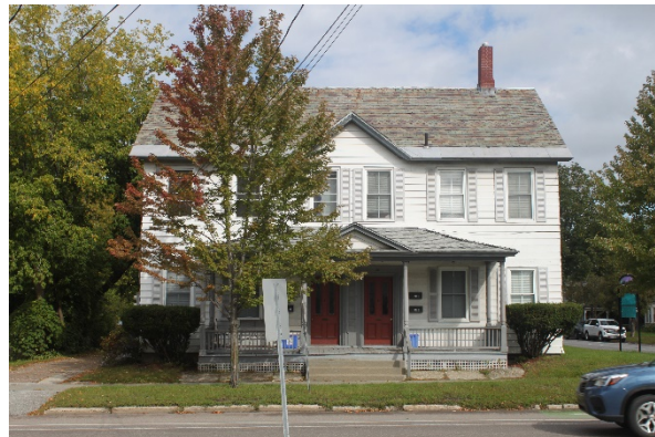
Figure 5 – entrance façade, 44-46 Sherman Street. View facing north. Taken by author, 9/26/2022
