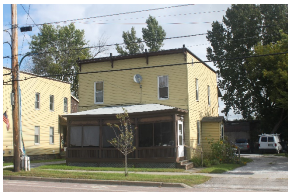
Figure 12 – 108 North Avenue, primary façade. View facing east, photo taken by author, 9/26/2022
