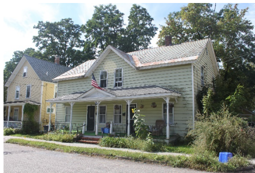
Figure 18 – 71-73 Lakeview Terrace, ¾ record shot showing depth. View facing southwest, photo taken by author, 9/26/2022.
