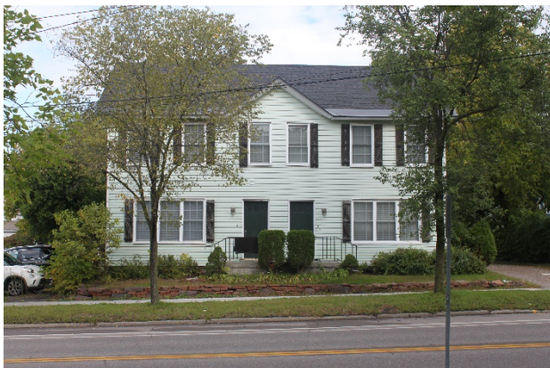
Figure 1- South façade of 30-32 Sherman Street. View facing north, picture taken by author 9/26/2022.
