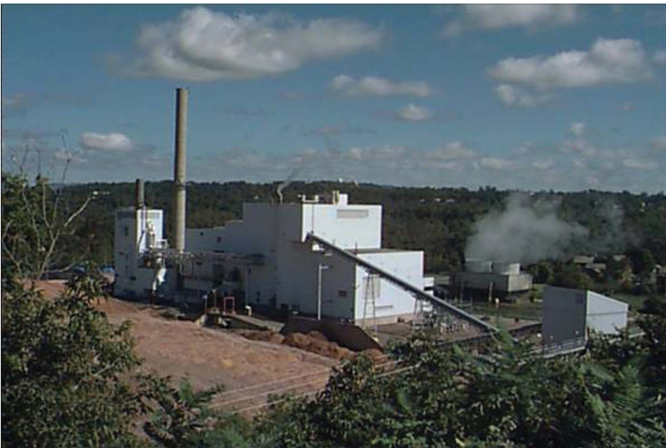
FIGURE 1 The 50-MW wood powered steam turbine McNeil Station, Vermont, USA (Source: Burlington Electric Department, 2011) (color figure available online).
