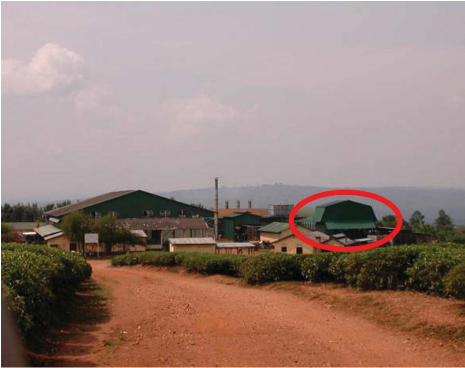
FIGURE 2 The 200-kW wood gasifier (circled) at Muzizi Tea Estate, Uganda (Photo: Buchholz, 2007) (color figure available online).
