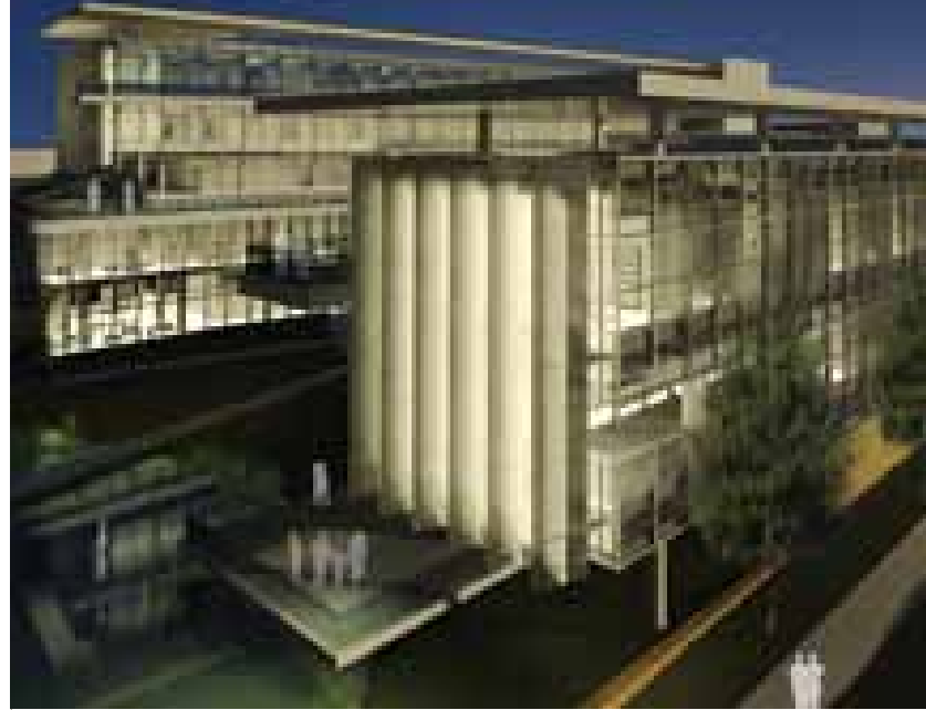
■ A new research building at the University of Florida, reflected in this rendition, will house the university’s Institute on Aging, focused on developing new research approaches to improve the health, independence and quality of life of older Americans, as well as the University of Florida Clinical and Translational Science Institute, a member of NCCR’s Clinical and Translational Science Awards program.
