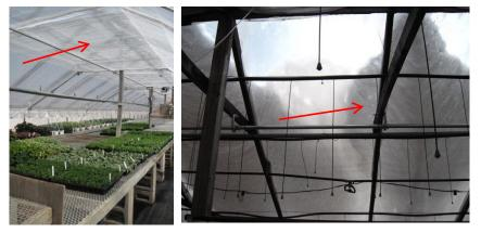
Left: Energy curtain (red arrow). Right: Soap bubble system in operation (red arrow indicates soap bubbles being generated)
