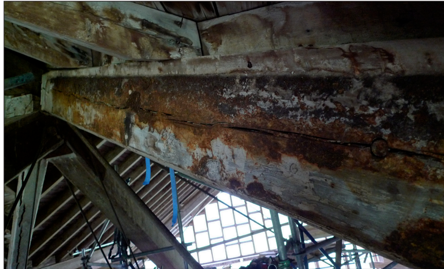
Steel channels left scaly rust deposits and stains on timber surfaces. Cleaning involved use of a nonionic detergent and water
