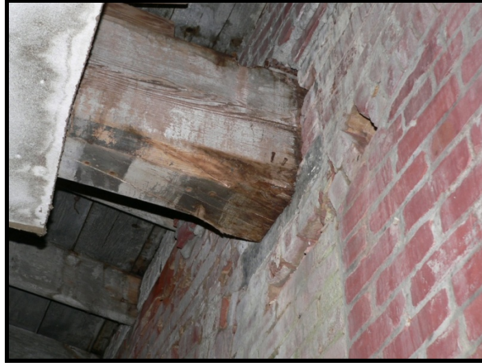
Unknown beam condition and bearing area within masonry wall
