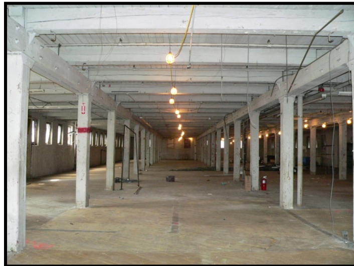
Beam-column-decking system with limited diaphragm action
