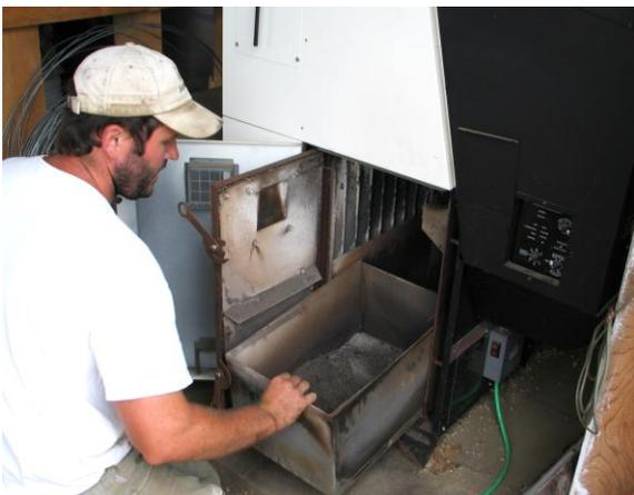
Kevin maintains the furnace carefully. "I give the heat exchanger a good cleaning after every ton, about 3 times a heating season, and I empty the ash pan, scrape the fire box and clean out the fines from the igniter box after each ton. This takes 30 to 45 minutes. At the end of the season a more thorough cleaning gets done including cleaning the combustion fan, the complete fire box, auger mechanism and the Sensor (the brains of the furnace). It takes two hours to do that well."
