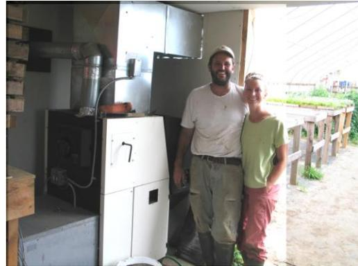
There is an HAF fan that circulates the forced hot air 12' (3<sup>rd</sup> bow) from the plenum outlet throughout the house. A second HAF fan is located at the other end of the house. The thermostat is located in the middle of the greenhouse 4' above the ground. The potting shed is insulated with 2" rigid foam (R-9 or R-11 value.)
