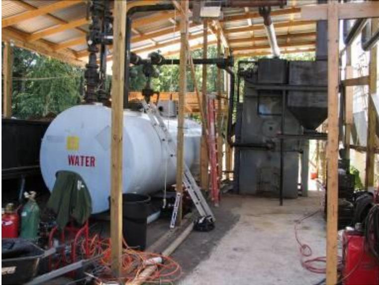
*The 3 million Btu Conifer furnace heats water in the Kewanee boiler; valves are set to control how much of the hot water is sent to heat the greenhouse or stored in the 3,000 gallon reservoir.*
