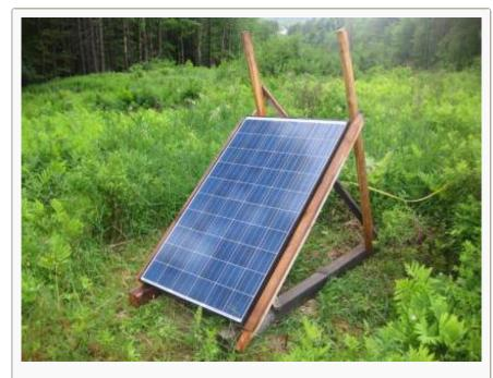
This panel is being used for water pumping. The wood-framed rack is simple and inexpensive, and can be adjusted to produce more power during seasons when the sun is lower on the horizon
