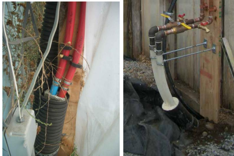
Figure 6 – A less expensive, less insulated flexible PEX product is shown on the left (FarmTek – Thermal Barrier @ $6.95/ft) and a more expensive, better insulated flexible PEX product is shown on the right (LogStar @ $18.00/ft). The cheaper option uses a foil bubble wrap with a manufacturer claim of R-value =1.1 per layer and the more expensive option uses expanded polyurethane foam with an R-value of 6 per inch.) In defense of the foil bubble wrap, it appears this is a poor application for the product. According to its manufacturer, it is intended to be a single layer radiant barrier, not a multi-layer insulation against conductive losses. The latter is what is needed to prevent underground losses.
