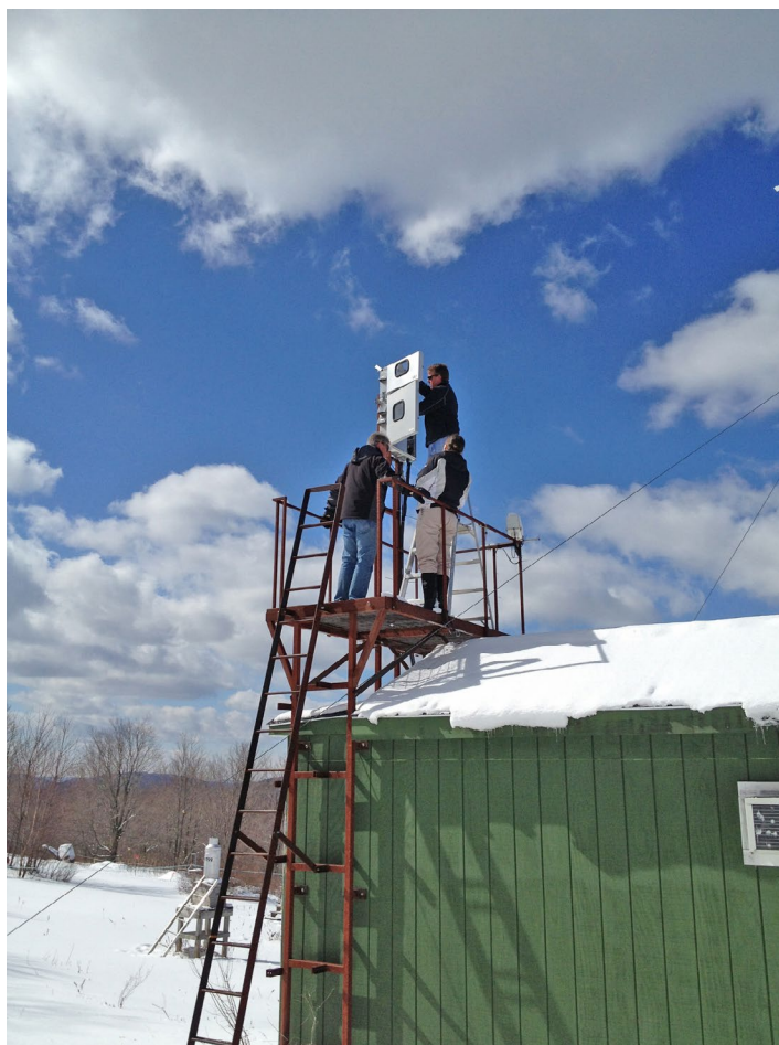
Mark Olsen demonstrating streamlined servicing of Tekran1135 particulate mercury speciation module.
