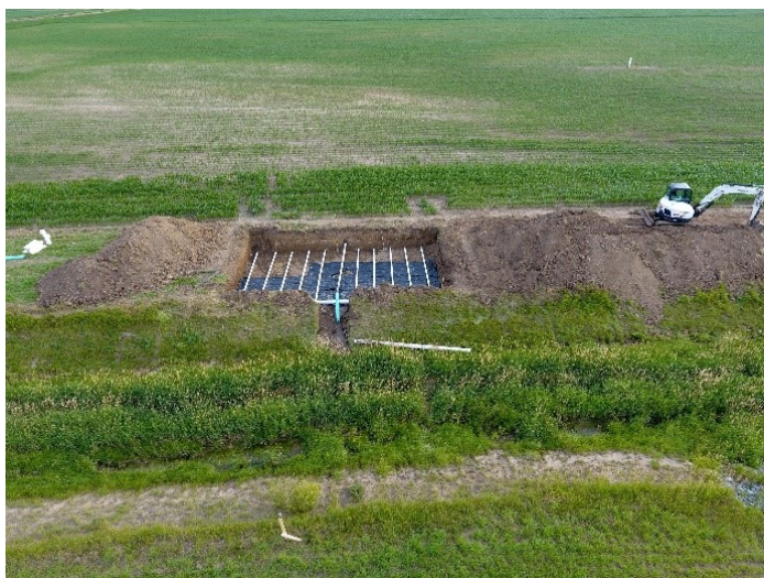
Figure 2. Installation of a phosphorus removal bed. (Photo courtesy of Blanchard River Demonstration Farms Network)
