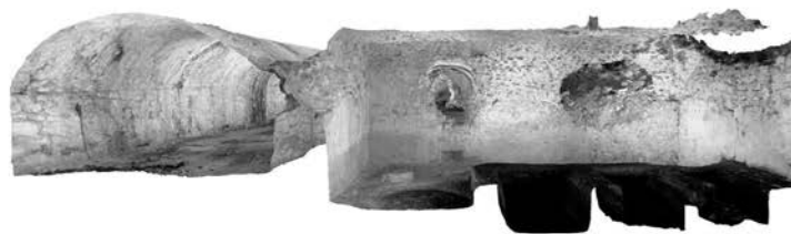
Fig.2/ Cross section from a perspective view of the main area of the cryptoprticus. The point cloud was transformed in a surface model through the meshing process.
