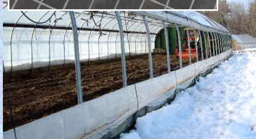
Curtains and corner panels to seal roll-up sides
