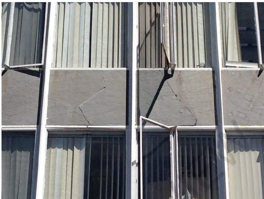
Enlarged view of the typical casement style steel windows and slate spandrel panels. In this view, the panels are exhibiting cracking
