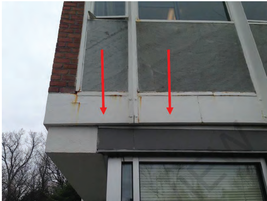
Exterior view of the Northwest building corners of McAuley Hall. Note the vertical deflection (or sag) observed at this location.
