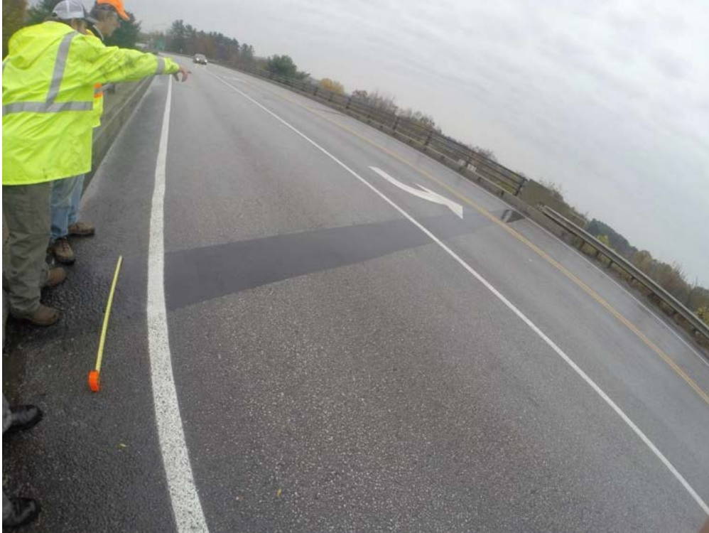
Figure 5.16 Rubber-asphalt expansion joint over abutment of Colchester/Milton I-89 Bridge
