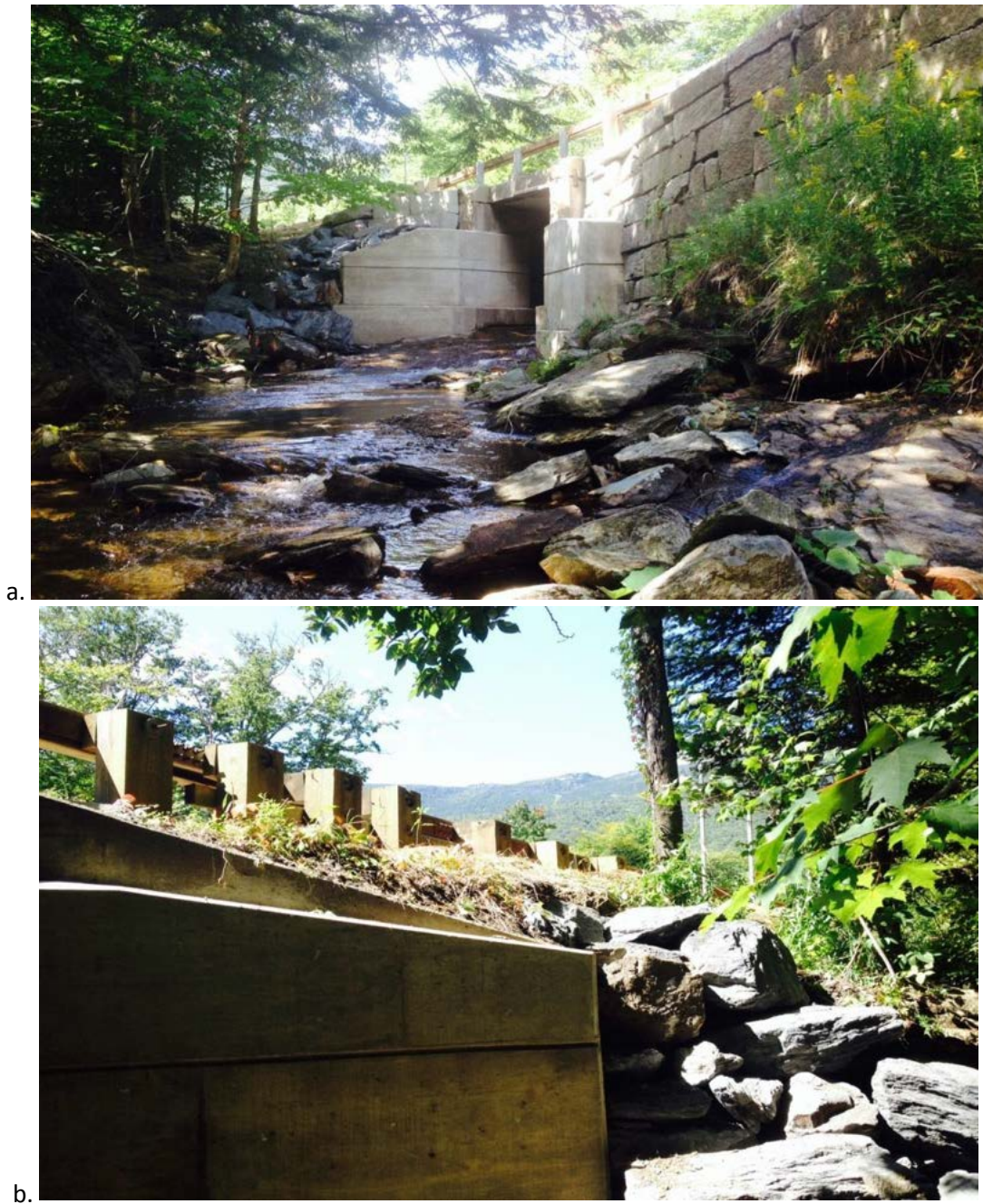
Figure 4.38 Vt. Rte. 108 Stowe Br. #10 – Repaired Wing Wall Encasement/ Other Repairs, $200,000
