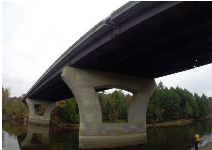
Figure 23: Bents, deck and beams
