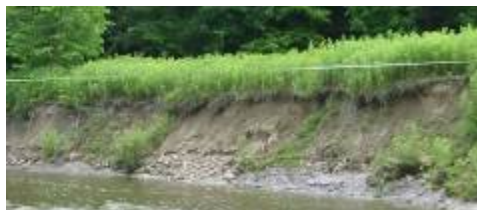
Figure 1: Example riverbank failure
