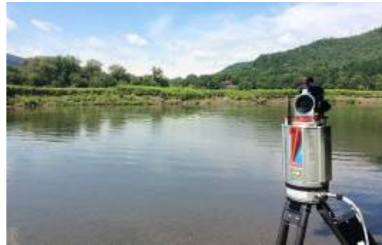
Figure 8. Streambank site along Winooski River with active erosion being scanned by the terrestrial LiDAR
