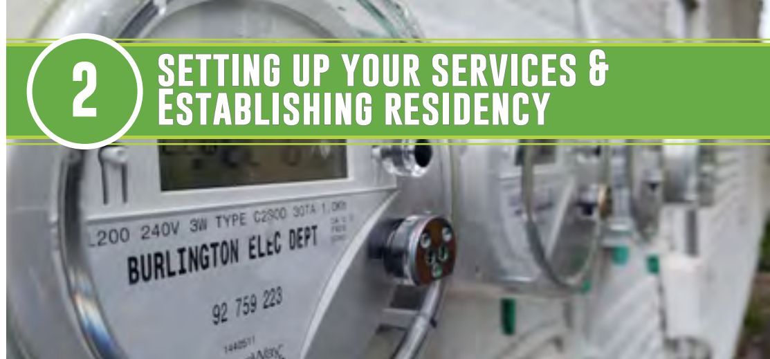
Collection of electrical meters for different apartments in the same building in Burlington.
