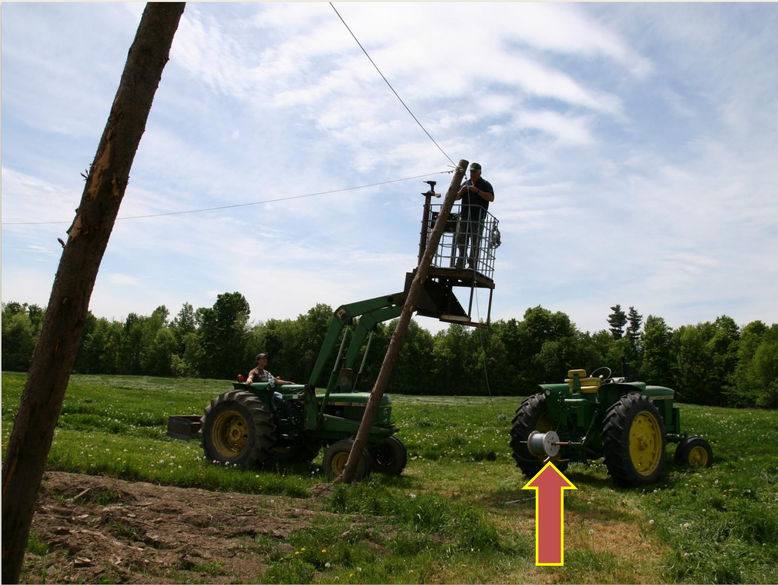
Cabling Hopyard Cable Spool On Tractor 3 Pt Hitch
