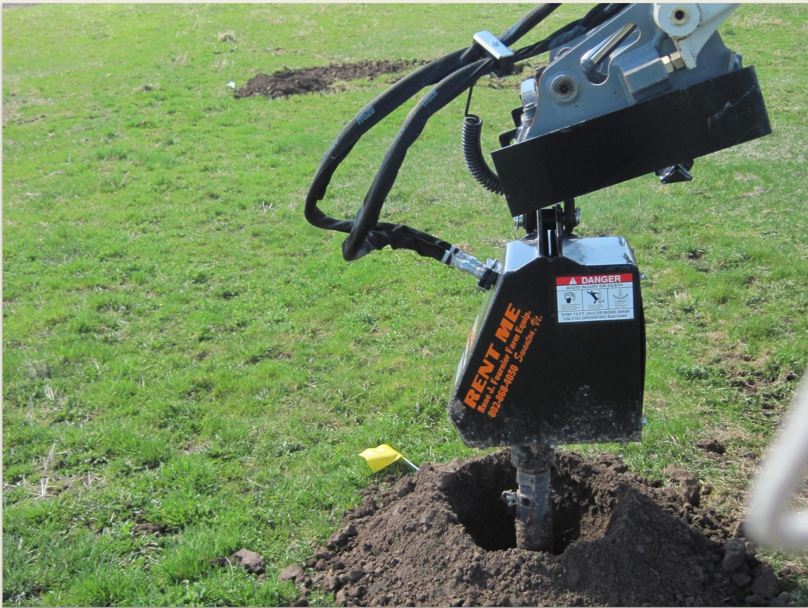
Drilling 4 Feet Deep to avoid Frost
