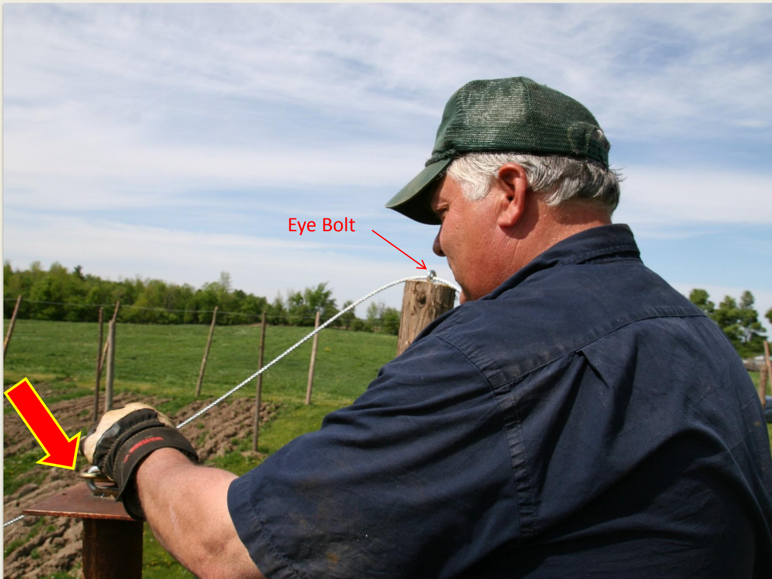
Hooking cable to haven grip to pull cable.
