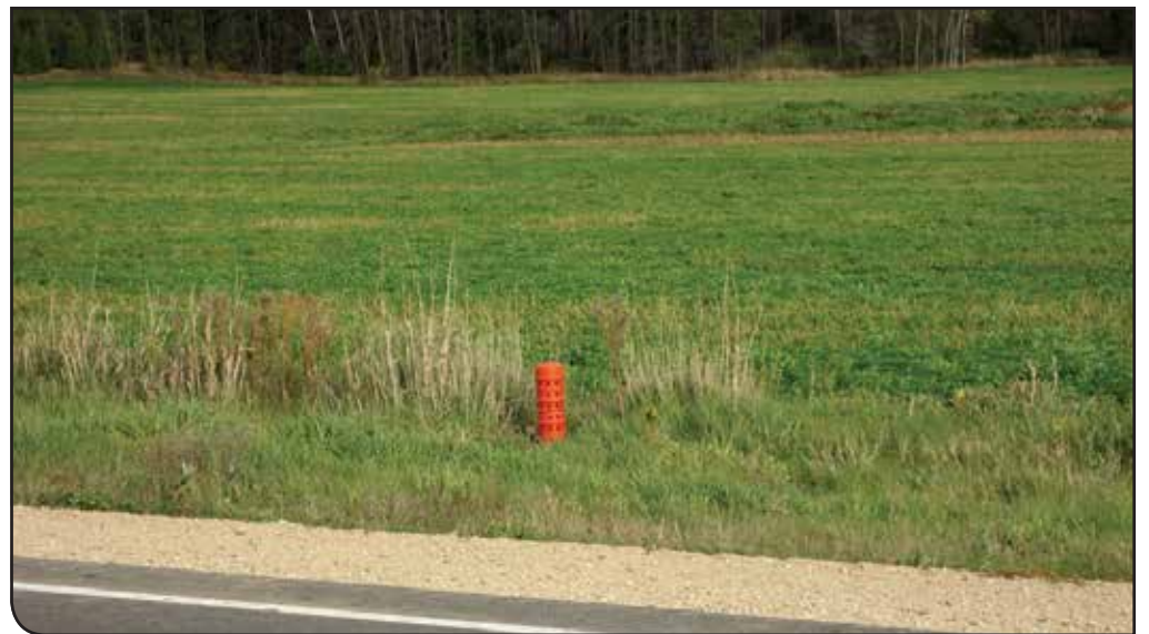
Figure 5: Tile vent installed at field edge.
