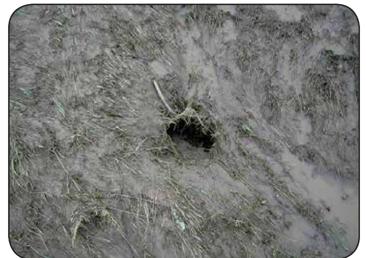
Figure 2: Sinkholes caused by tile blowout.
