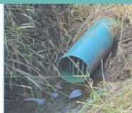
Figure 1: Tile outlet with a rodent guard.
