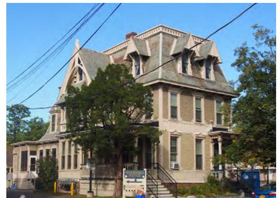
MARTIN L. KELSEY HOUSE, 43 ELMWOOD AVENUE
