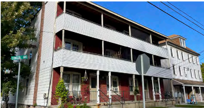
29-33 CONGER AVENUE, LOOKING NORTH-WEST AT PRINCIPAL ELEVATION
