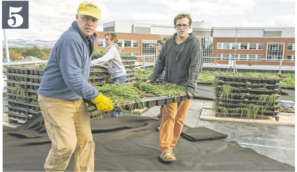
5 Research associate Gary Hawley worked with students to move the plants to their designated spots among the watersheds. Students have been an important part of the process, contributing ideas during the design phase as part of the "Greening of Aiken" course and providing much-needed muscle to move the 120-pound flats to their proper locations during the installation.
