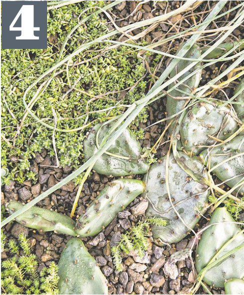
4 The roof will test the effectiveness of different species of plants and types of soil at absorbing stormwater and keeping pollutants out of surrounding watersheds.
