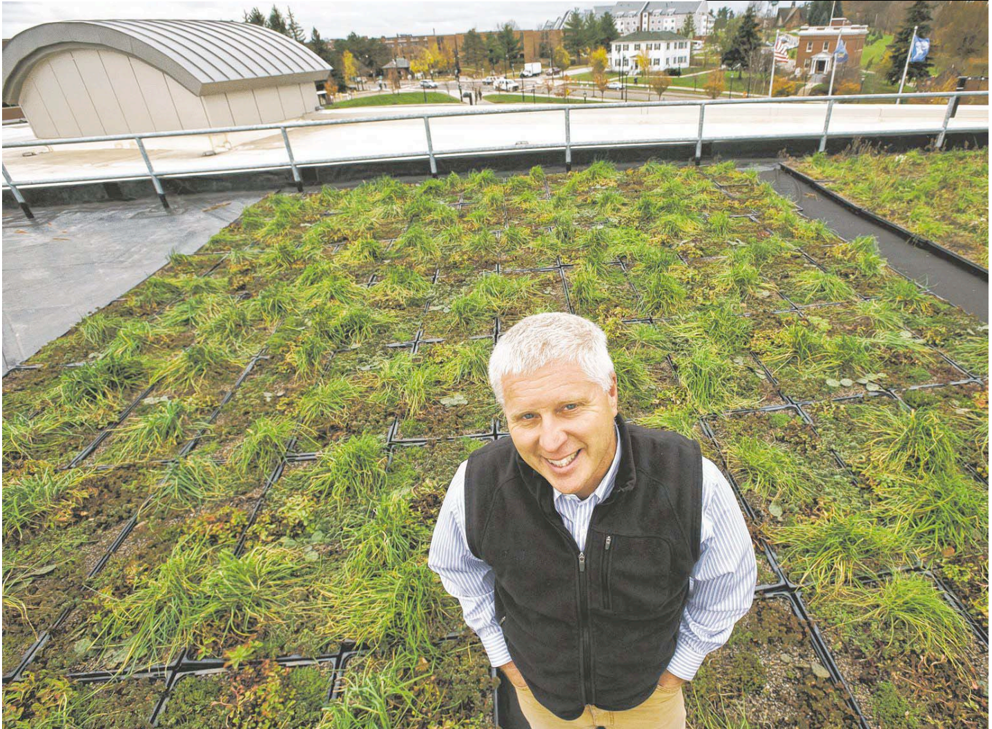
Gary Hawley on the green roof at the Aiken Center at the University of Vermont in Burlington on Thursday. GLENN RUSSELL/FREE PRESS
