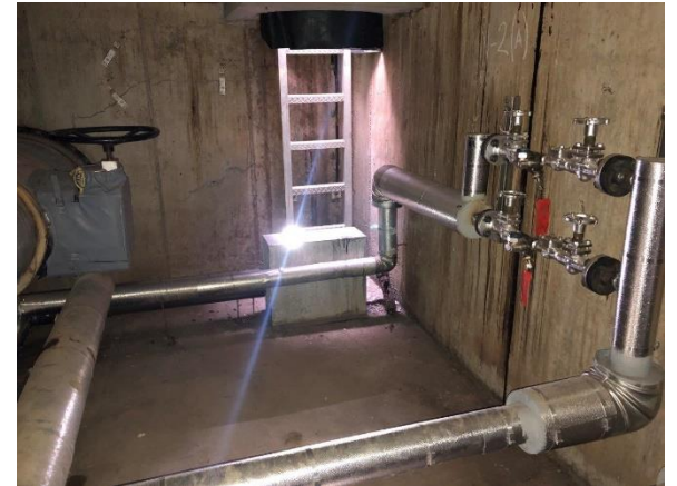
42 steam and chilled water vaults are getting repaired.
