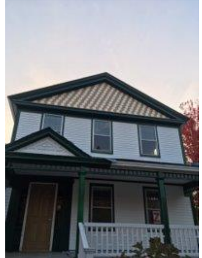
Wadhams House project scope included foundation, storm windows, wall insulation and a new roof.
