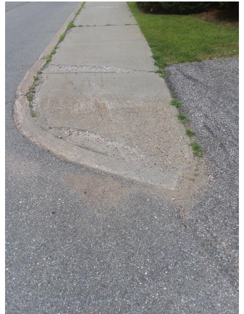
Delahanty – Fix the grade and concrete
