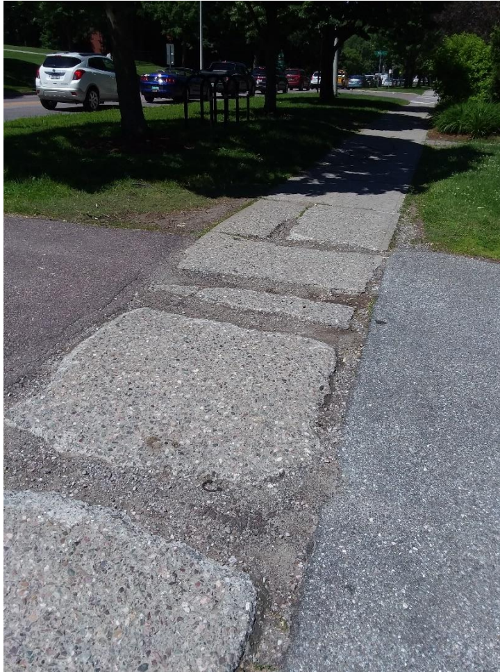
Jacobs House – Redo the sidewalk
