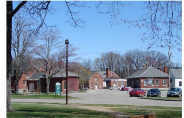
3. Looking north to Physical Plant buildings on the right
