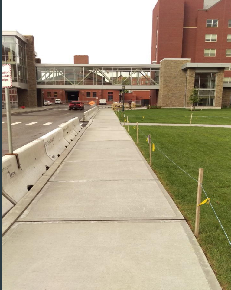
6' Walkway to Central Heat Plant
