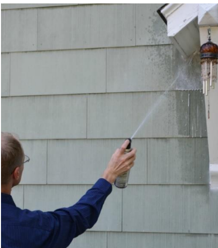
Spraying from a distance in a wall void.
