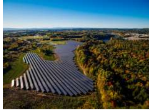
Figure 27: solar panels in an array in Williston. Photo provided by Green Mountain power.
