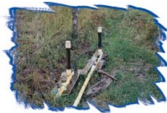
Twin ram pumps.
