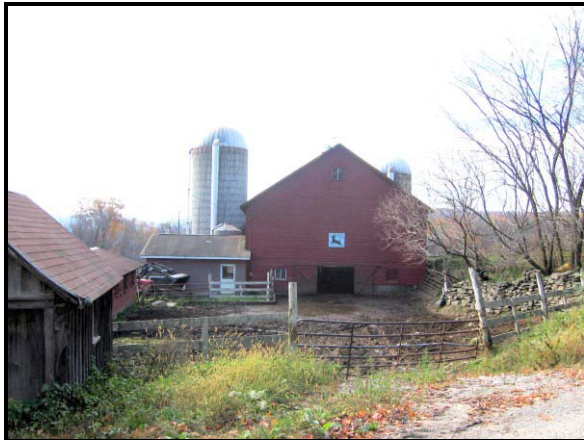
Main Dairy Barn
