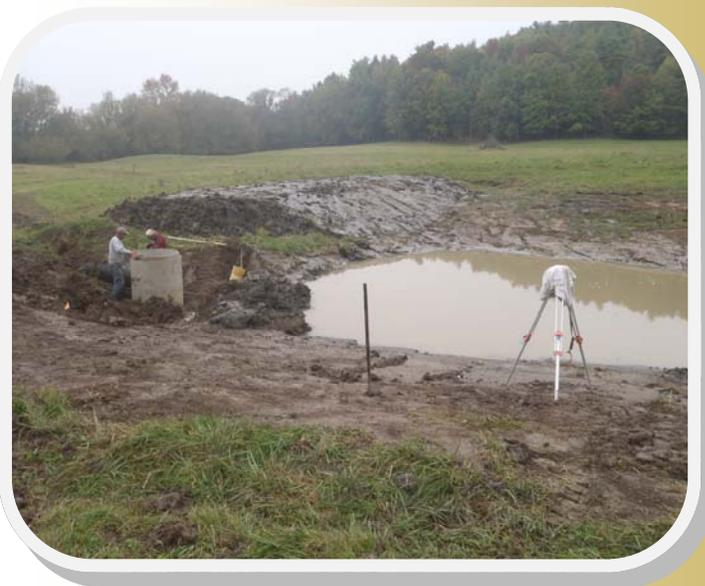
Pond berm was rebuilt with overflow and water intake structure for gravity fed water system.
