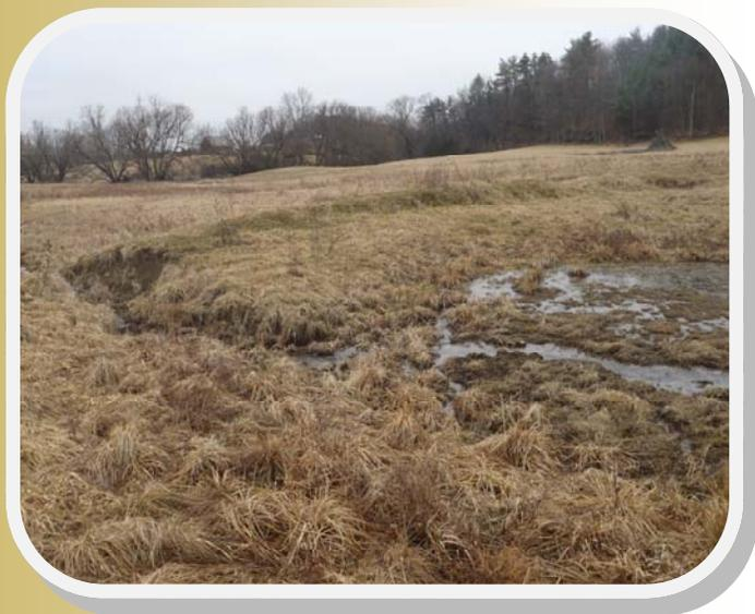
The berm of this farm pond failed, leaving no water source for livestock.
