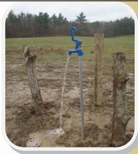
Water lines installed under the new berm supply two frost hydrants. Clean water for livestock and the lake!
