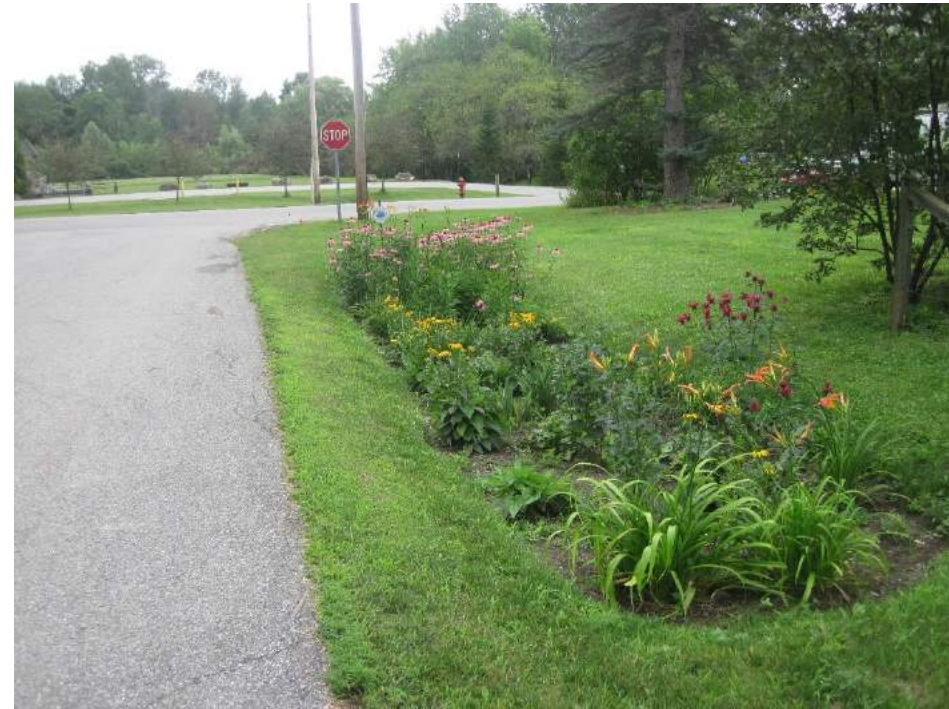
Swale with Raingarden, Woodbine Road, Shelburne, 2017
