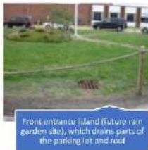
Catchbasin which drains directly to McCabe's Brook, untreated.
