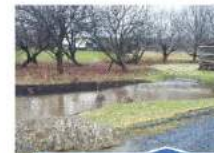
Example of water being contained in a bio-retention area after rain event.
