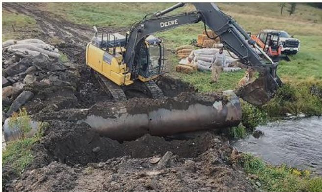
Ski lift tower culvert removal on Valley Brook.
