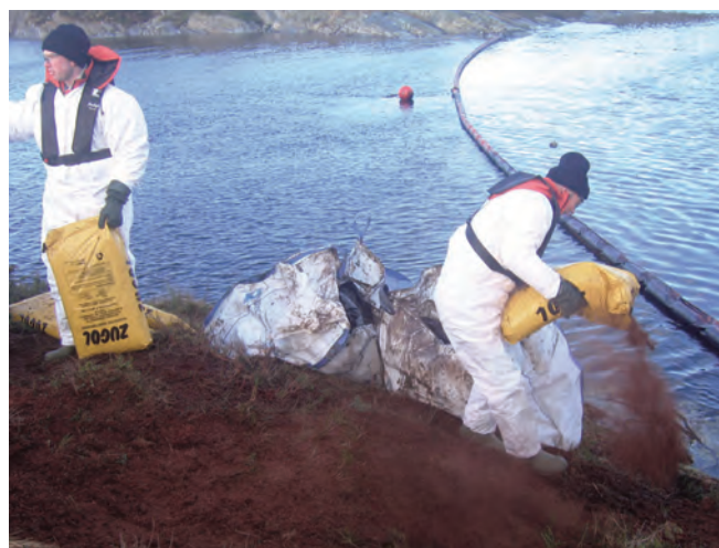
▲ Figure 10: Organic particulate sorbent material such as peat or bark may be applied on rocky shores of importance to wildlife (e.g. penguins and seals), to minimise contamination to fur and feathers as they come ashore.
