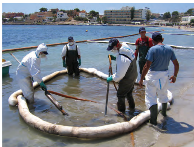
▲ Figure 1: Polypropylene sorbent boom used to collect oil released during flushing operations.
