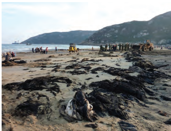
▲ Figure 13: Sorbent pads stranded on a shoreline at high tide, after deployment at sea. Unless removed quickly, sand movement during subsequent tides will cover the pads, hindering recovery.
