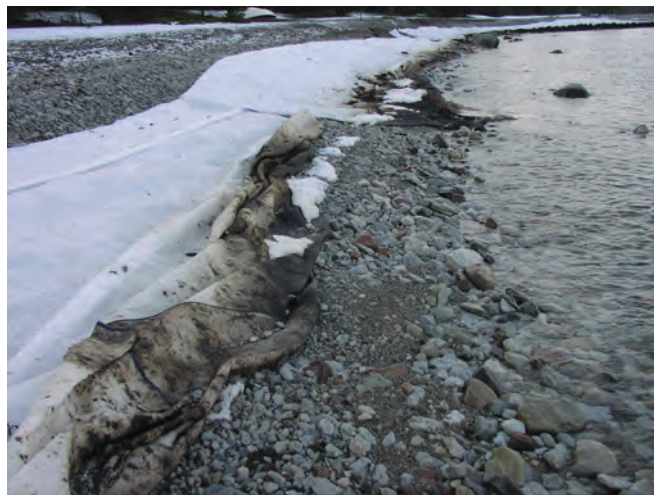
▲ Figure 5: Continuous flat sorbents, such as this sheet laid on a shoreline, are characterised by a high surface area to volume ratio. The large scale use of sorbent in this manner should be balanced against the generation of considerable volumes of potentially unsoiled waste.
