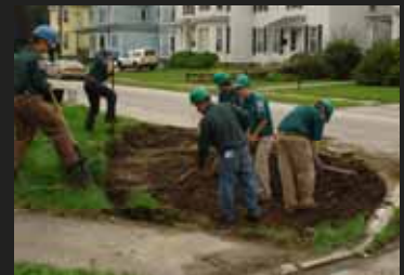
Build next to a road
