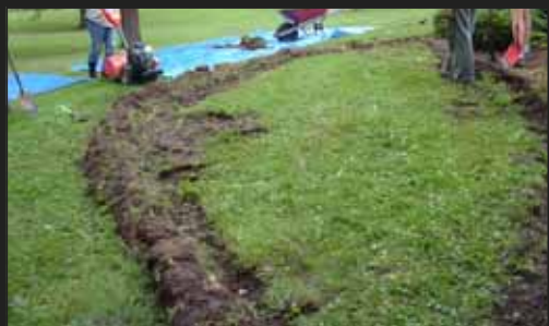
Build the berm with sod
