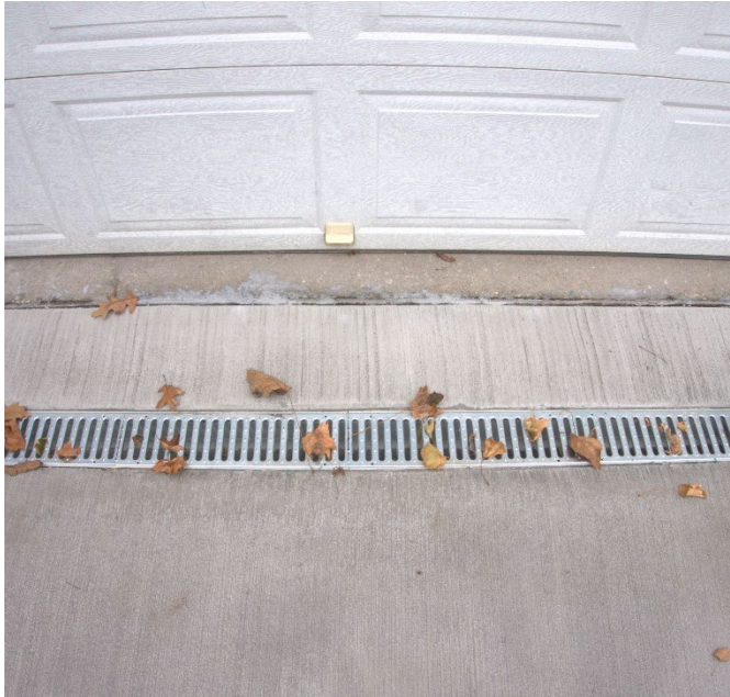
[Above] Driveway trench drain connected to a backyard dry well.
