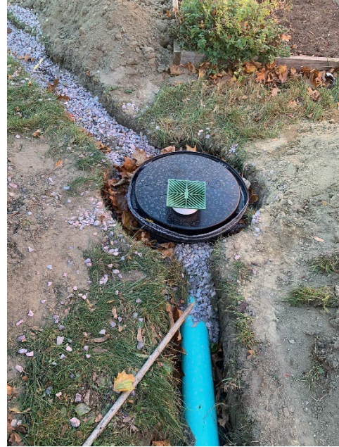
[Above] Driveway trench drain connected to a backyard dry well.
