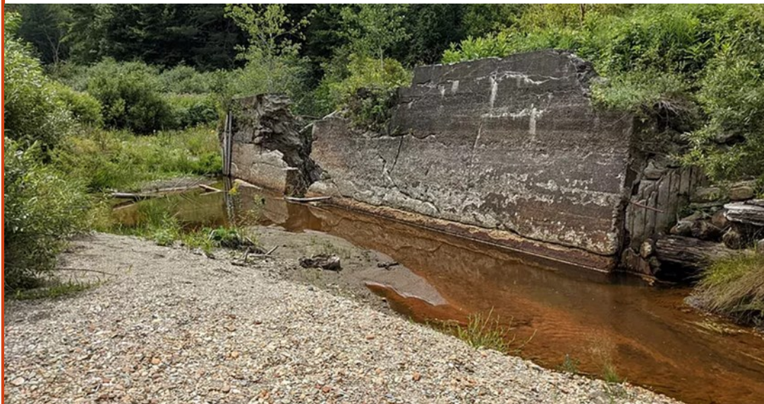
Above: Dam before removal (looking downstream). Breached portion in center of dam.
