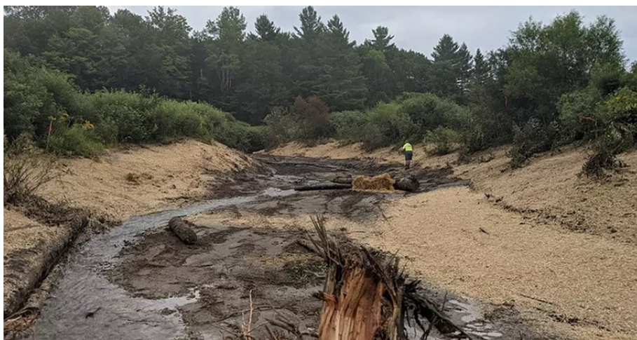
Below: Bogue Branch channel and streambanks following channel restoration and bank stabilization work (looking upstream). Banks to be planted with live willow stakes in fall 2021.
