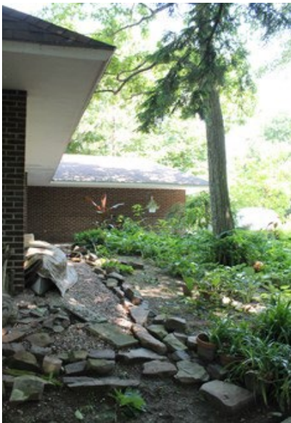
[Left] Roofline infiltration trench. [Right] Impervious surface removed and replaced with vegetation.
