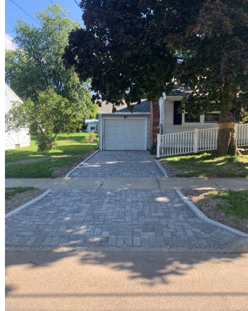
[Left] Impervious surface removal replaced with stepping stone path. [Right] Permeable paver driveway.
