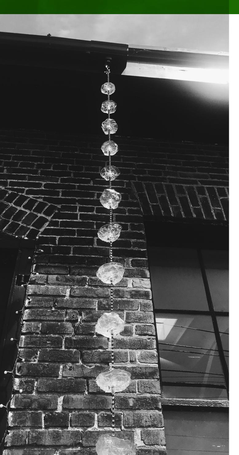
Here on Pine Street, rainstorms often cause flooding and carry pollutants to Lake Champlain from pavement and rooftops. Each year, the roof of an average size home in Vermont will capture and shed nearly 45,000 gallons of rainwater! RAIN CHAINS like this one reduce stormwater runoff by directing stormwater from roofs to lawns and other permeable surfaces, where it can be absorbed.
