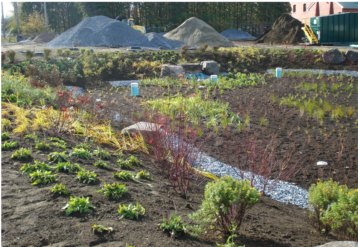
Gravel wetland installation at Burlington's Waterfront Park. Credit: Rebecca Tharp
